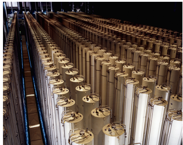
Dual-use item: Cascade of gas centrifuges to produce enriched uranium U.S. Department of Energy
